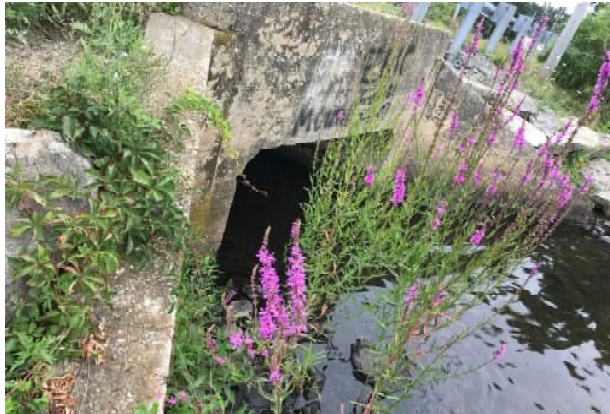
Figure 2A Route 58 Culvert (West Monponsett Pond side)
