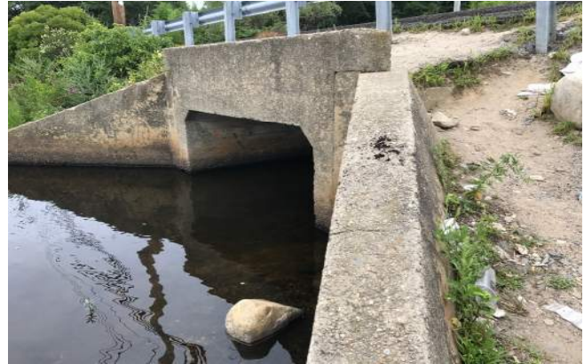
Figure 2B Route 58 Culvert (East Monponsett Pond side)
